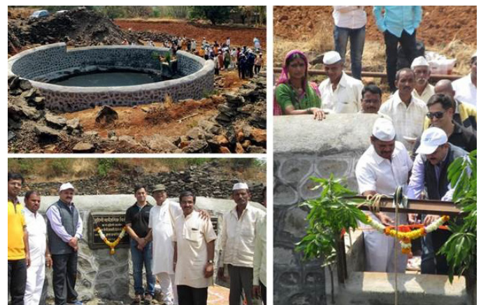
Well Excavation and construction at Guhini village, Pune
